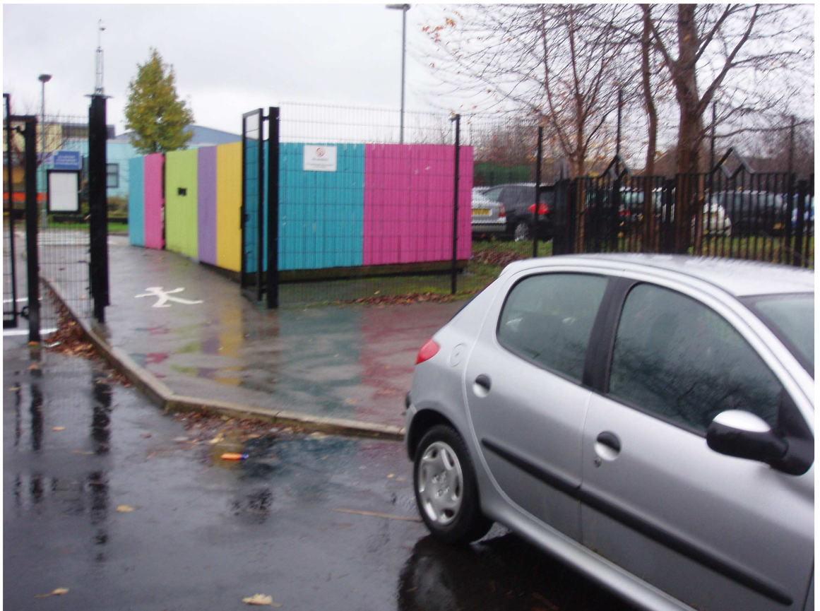
The build out outside the school entrance on the western side of Nottingham Street. Taking this new feature into account, it is proposed that double yellow lines cover the build out area only (a 5.6 metre length)
